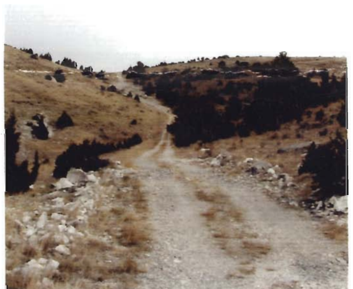
8 South View Approaching Drainage Crossing
