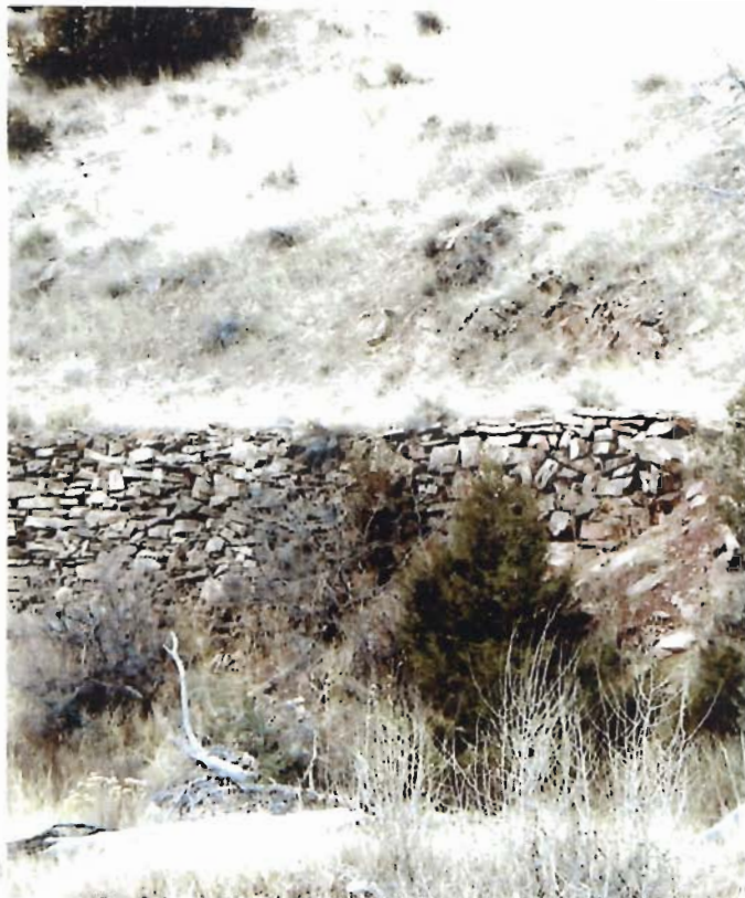
3 North Entrance Hillside Wall From Drainage
