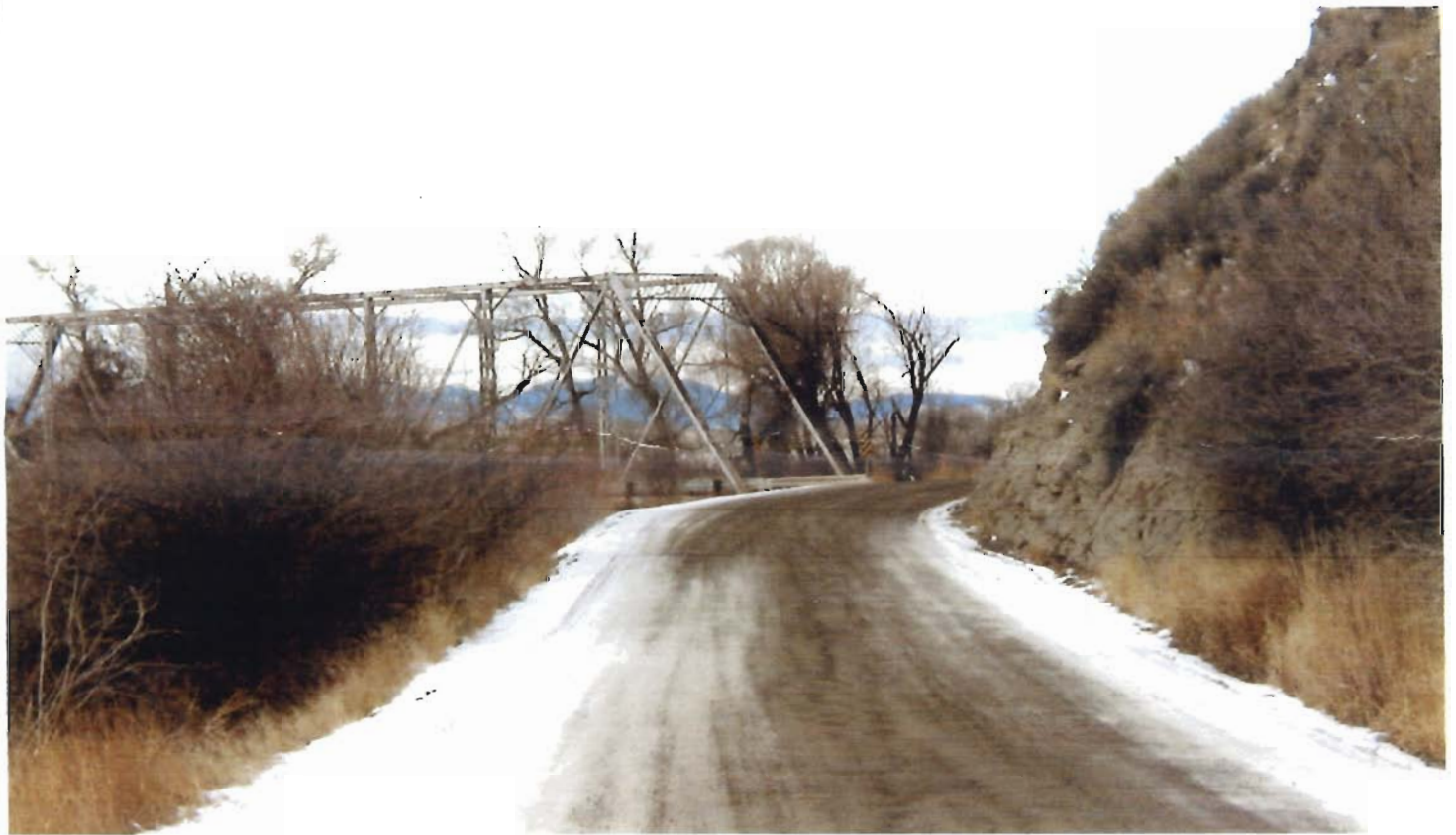
38 View of Cliff and 80 Degree Turn To Bridge
