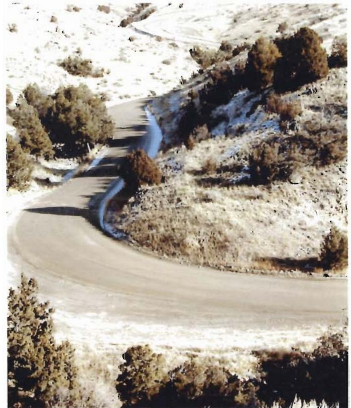
34 View of Hairpin in 33 Looking North
