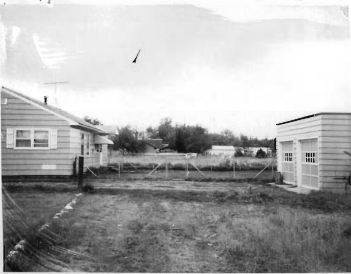
Looking So. on alley from NE corner lot 64
